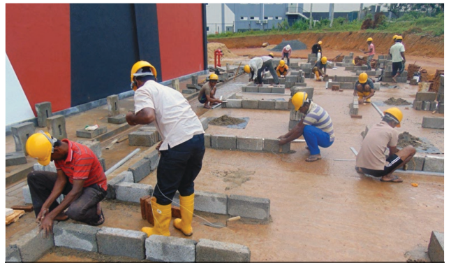
Competency Based Training Programme - Starting of Cement Block Masonry
