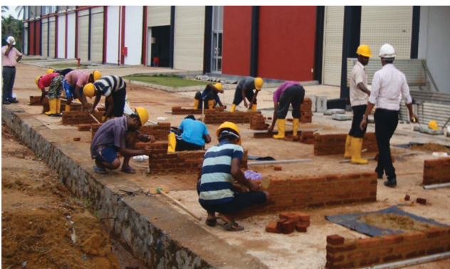
Competency Based Training Programme - Brick Work Masonry for 4 1/2" Stretcher Bond
